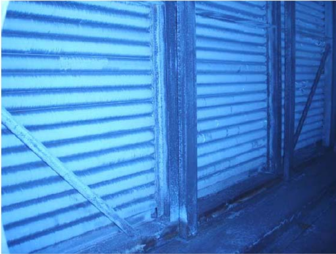
View of the FD Air side of the heater – showing the finned tubes, this is the outlet side of the heater as viewed from the front left lower man access door
