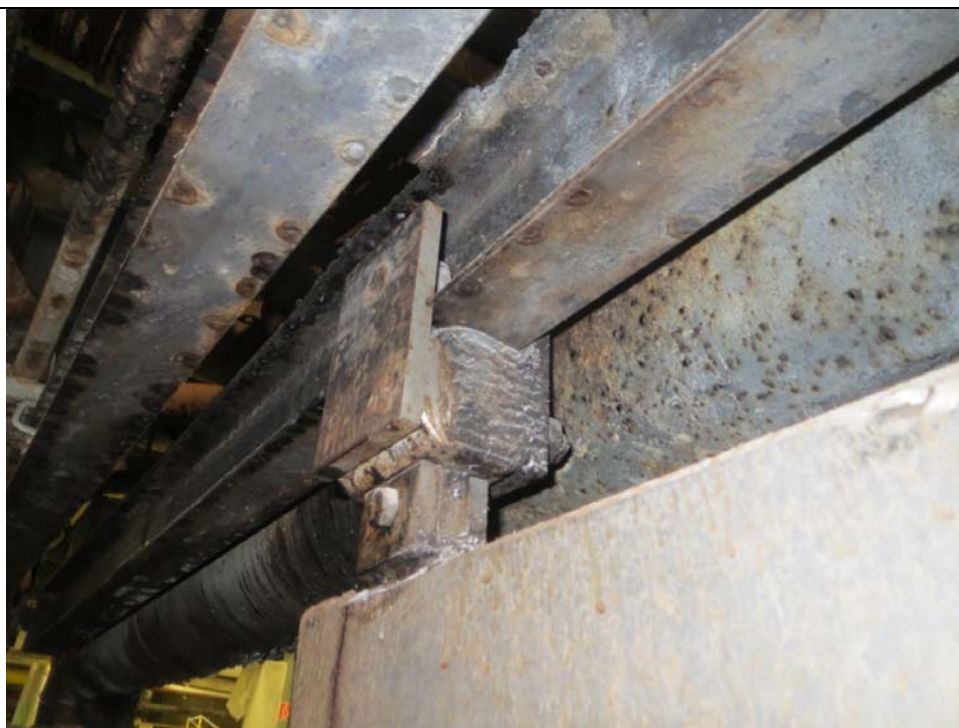
Movable Smelt Spout Shields on Track System
