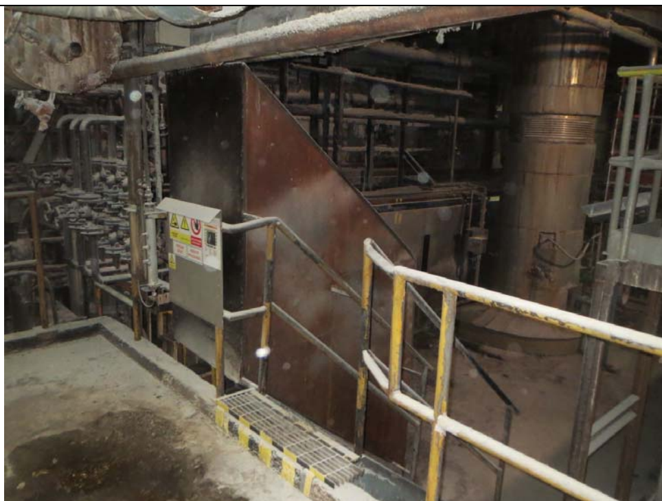
Shielding at Stairway Entering Smelt Spout Area
